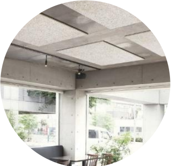
Acoustic Ceiling Panels
