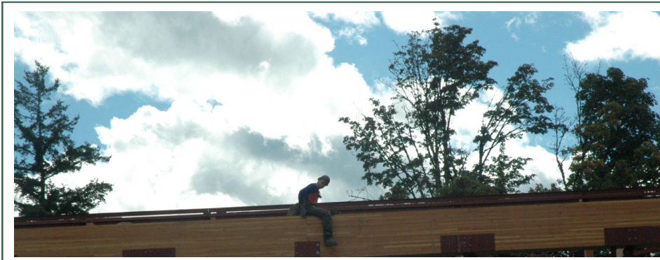
Busy, busy, busy — Construction at the new Canada Education Park
