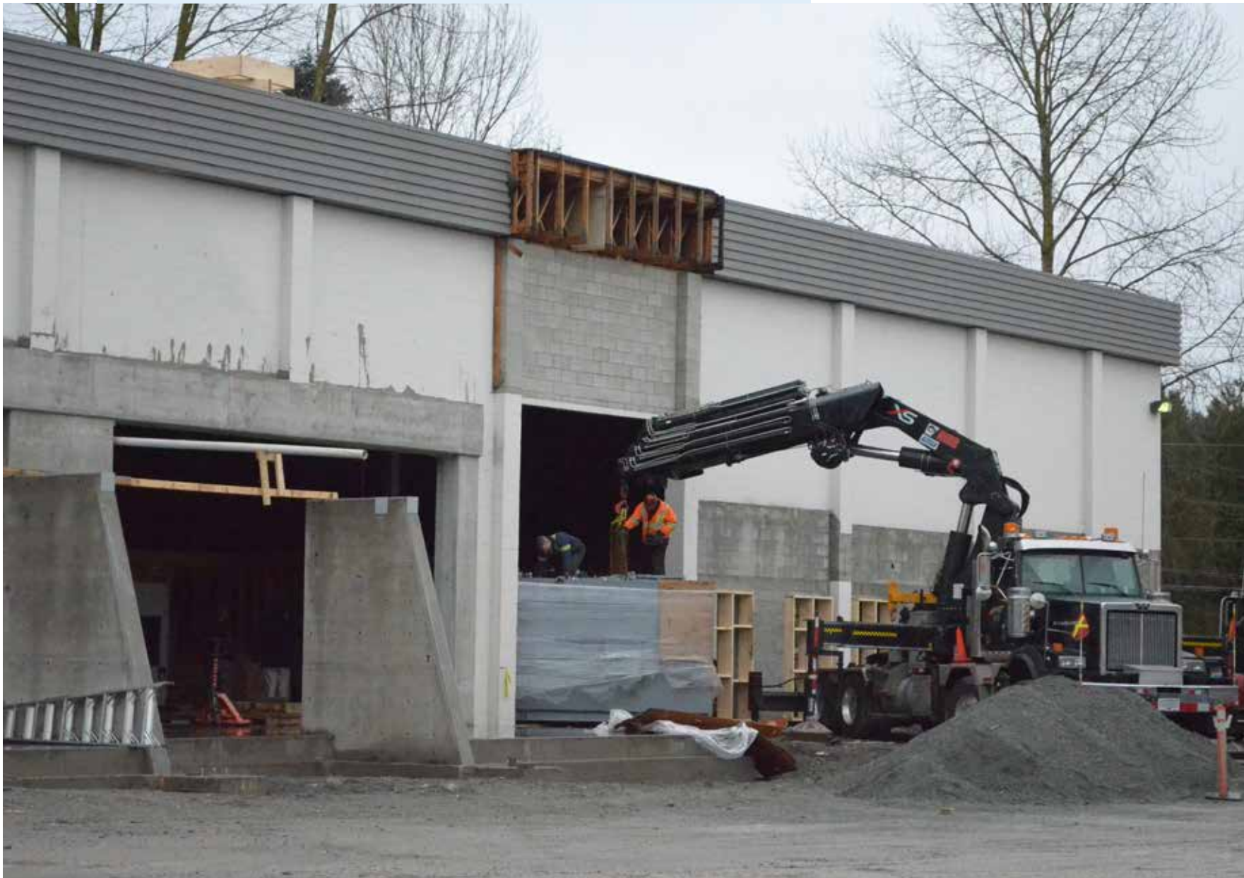
A crane unloads a retort into the building.
