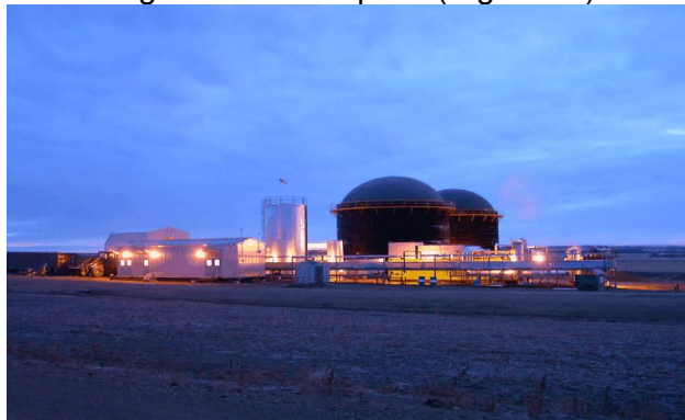
Figure 16- IMUS plant (Highmark)
